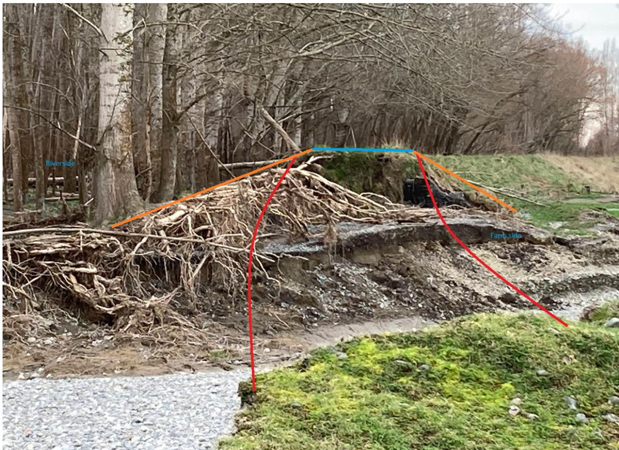
Figure 2: Section of washed out stopbank. The longitudinal crest followed the red lines, and the stopbank profile is shown by orange and blue.
