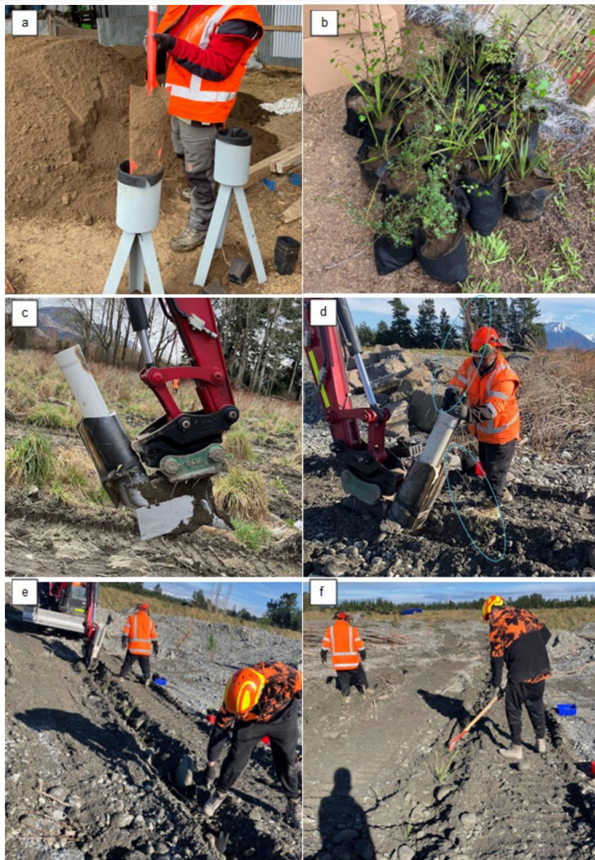
Figure 5, Terrafelt bag planting process. a) filling bags in custom tri-pod stands; b) filled bags with plants; c) the custom ripper; d) two ribbonwood trees being planted (circled); e) ripper row in progress; f) tidying around planted plants.
