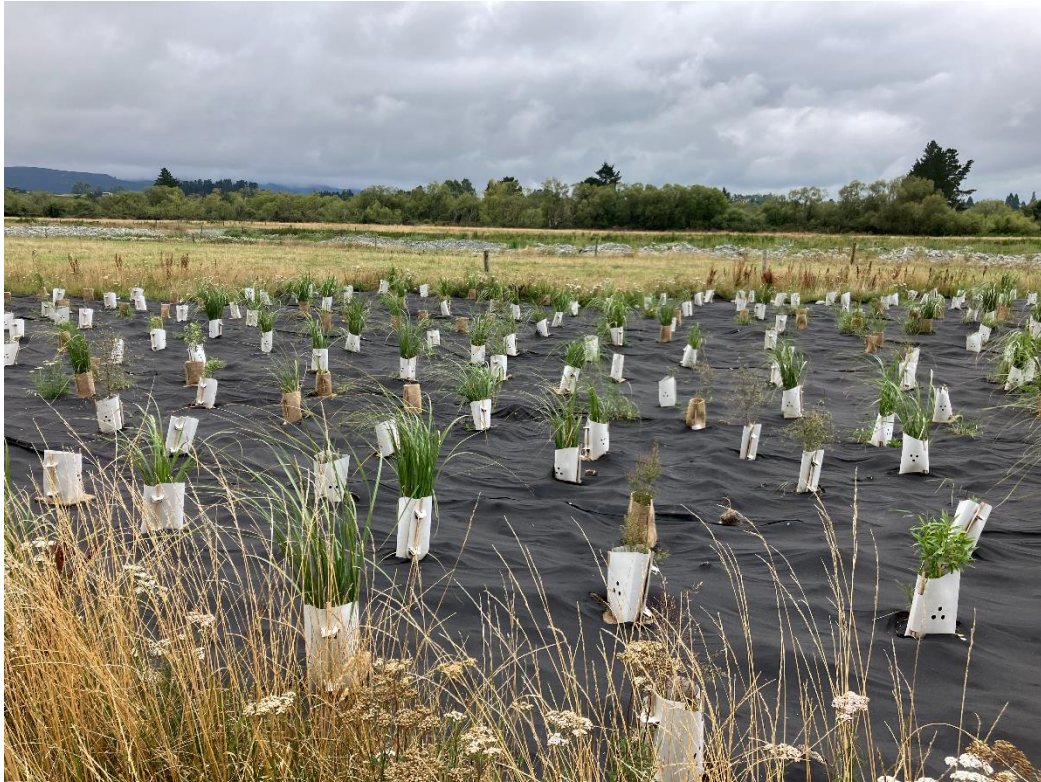
Figure 3, Extensive Terrafelt installations on the true right bank of the south branch Ashburton near Mt Somers
