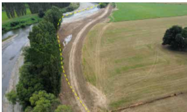
One of the three sections of stopbank replaced on the Waihi River at Hawke Road. The previous (destroyed) stopbank alignment is indicated by the dashed yellow line
