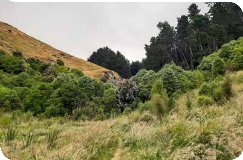
Well established planting at the Albert Stream site provides sediment filtering and shade for the stream
