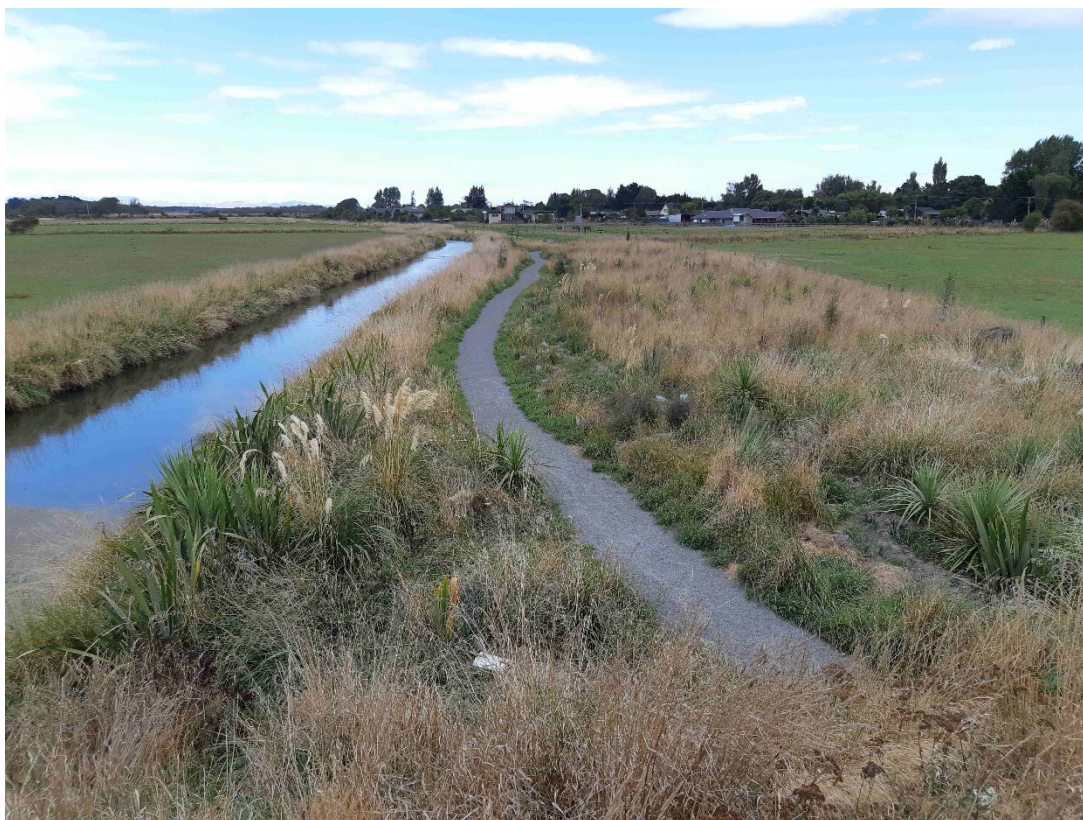
Figure 4: A crushed rock path was installed in 2019-20 for planting access and amenity along the Taranaki Stream Reserve.
