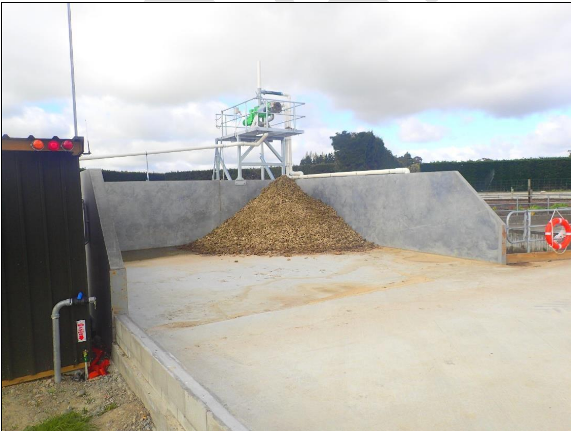
Figure 4 New solid separator installed in 2018.
