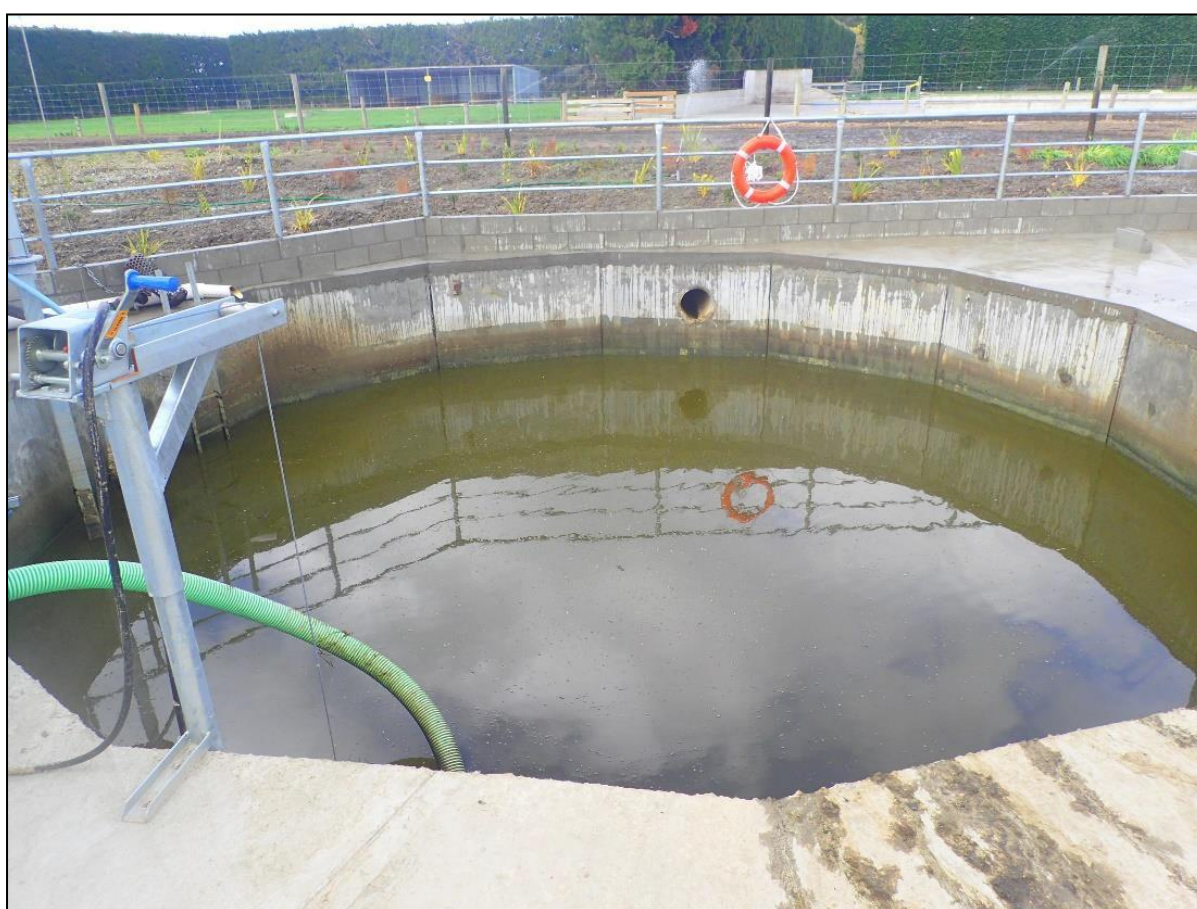
Figure 2 Upgraded effluent sump installed in 2018 and native plantings.
