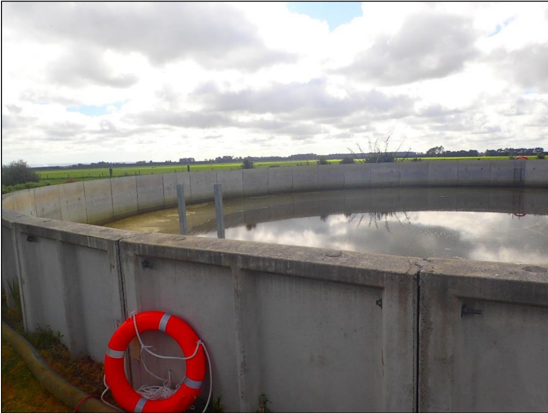
Figure 3 Updated effluent storage pond installed in 2012.
