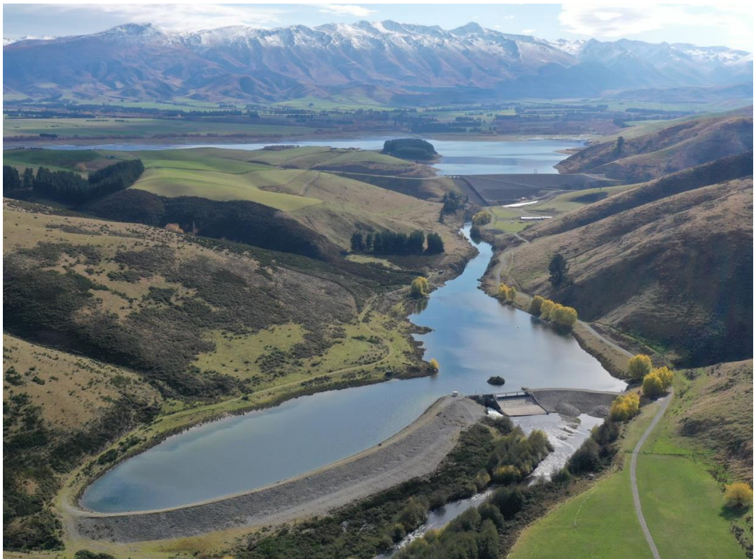
Figure 2. The Opuha dam, regulating pond and downstream weir (looking upstream).
