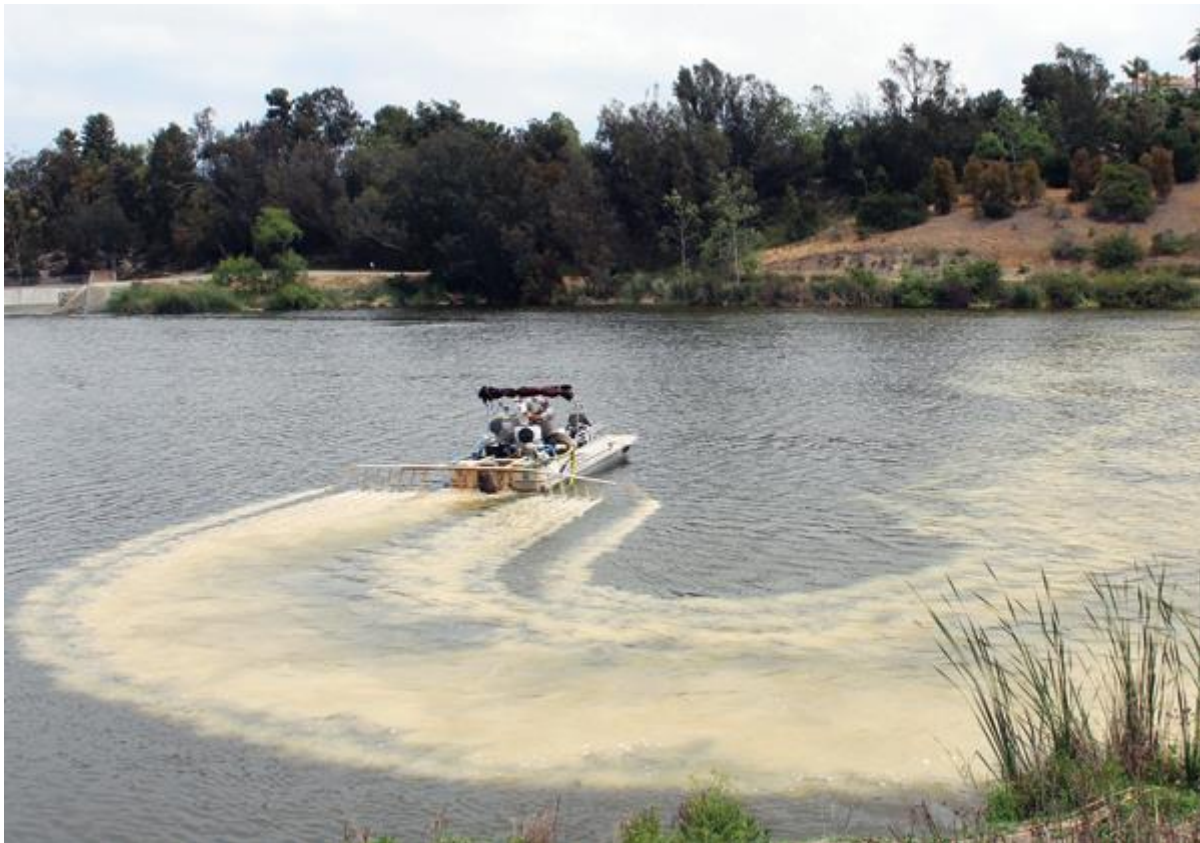
Figure 19: Example of full-scale Phoslock® application in a lake.
