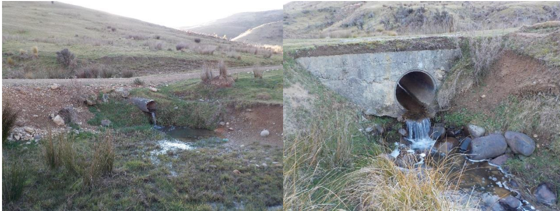
Figure 5: Perched culverts along Bush Gully.
