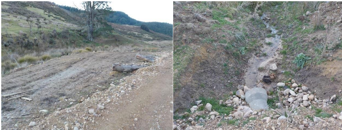
Figure 8: The access road and cleared ground (left) and channelised and culverted tributary (right).
