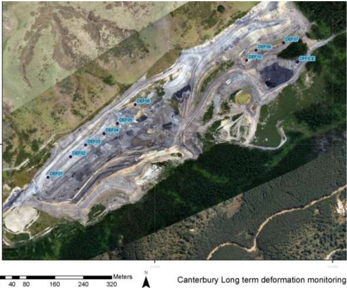
Figure 2: Canterbury Coal mine long term deformation survey markers installed 1 st July 2013 to record potential ground deformation within the footwall (DEF01-06), overburden tips/ELF area (DEF07-10) and site office
