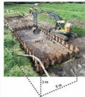
Figure 3. Finishing emplacement of reactive woodchip/gravel mixture into the first cell of the denitrification wall, which is oriented perpendicular to the direction of groundwater flow (from the left in the photo). The 50/50 binary mixture of wood and gravel was prepared on a volumetric basis and deposited into a dry excavation. Note: the sheet-piling was removed once the cell was filled. Denitrification wall dimensions are marked.
