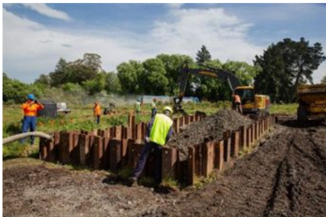
Construction of the denitrification wall using a mixture of woodchip and gravel.
