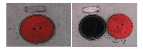
Lift the lid and locate the outlet valve. The valve will need to open, this can be found below a red toby (or lid) as pictured on the left.
