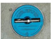
Firstly, lift the lid and locate the outlet valve. The valve can be found below a blue toby (or lid) as pictured.
