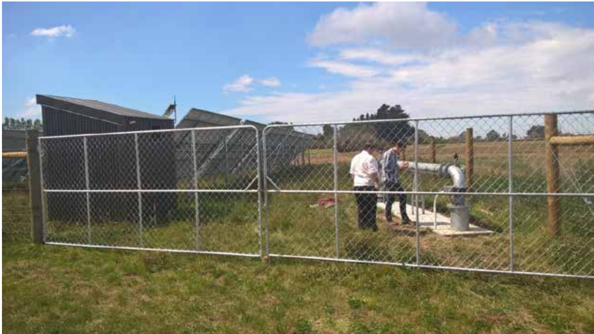
Figure 2. TSA Project site infrastructure components
