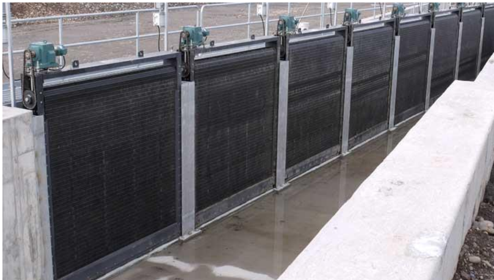
Figure 2: Example of travelling screen (Fall River, Hydolox screen)
