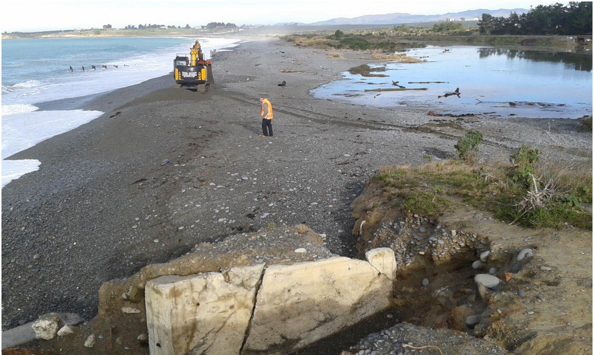
(Photo above shows start of mouth-opening excavations on shingle ridge in early July 2017, looking south. Concrete in foreground is reportedly from the structure of a former shingle processing plant. Below, the outflow begins in excavated channel.)
