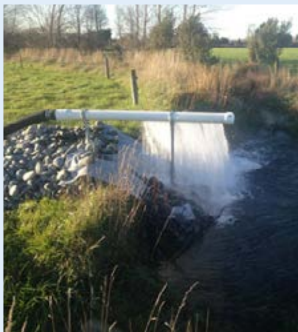
Water from a groundwater bore is used to restore water to a dry reach of Boggy Creek.
