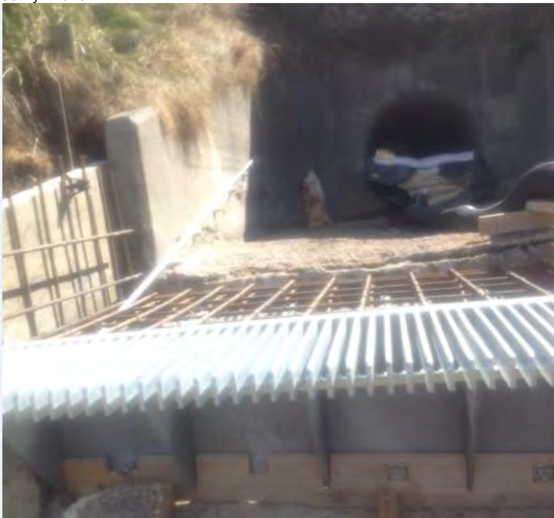
Below: Remediation works (trout barrier) currently underway at Coach Stream culvert, Selwyn Zone
