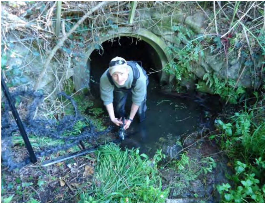
Above – Biodiversity Officer Rob Carson-Iles installs mussel spat rope to assist fish passage at a Waipopo culvert.
