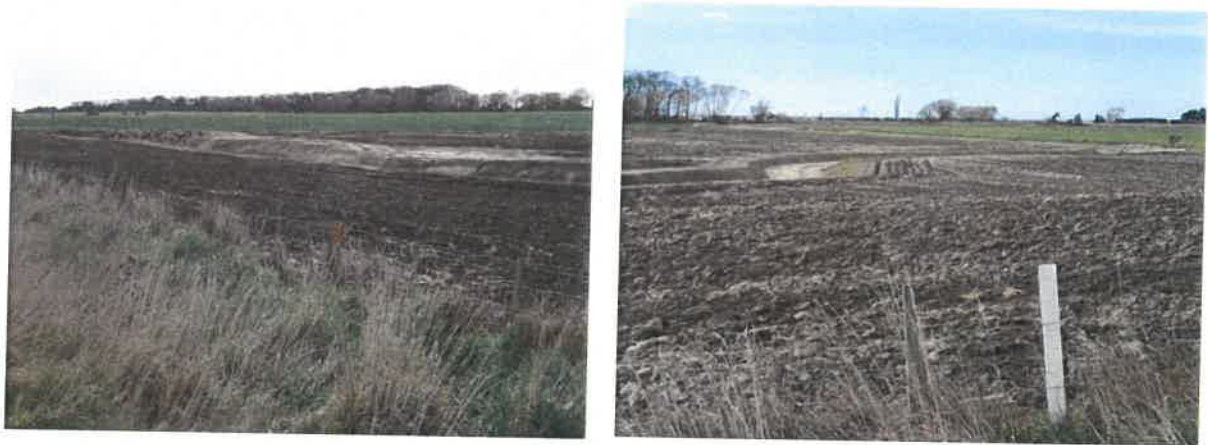
Figure 3. The reach downstream of Wallaces culvert, showing the realigned channel, re-contoured bed and banks, and lack of a set back to the cultivated ground. Photos by N.R. Dunn.
