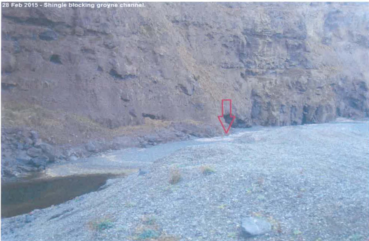
28 Feb 2015 - Shingle blocking groyne channel.
