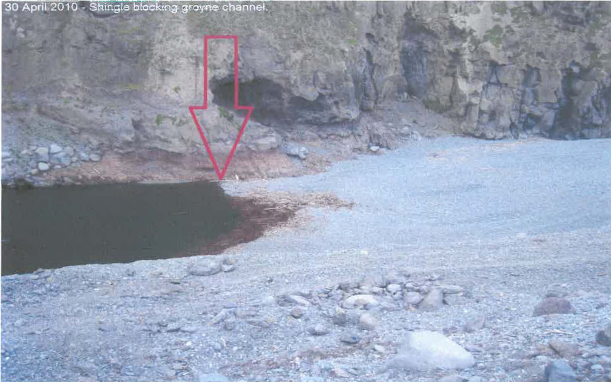
28 Feb 2015 - Shingle blocking groyne channel.
