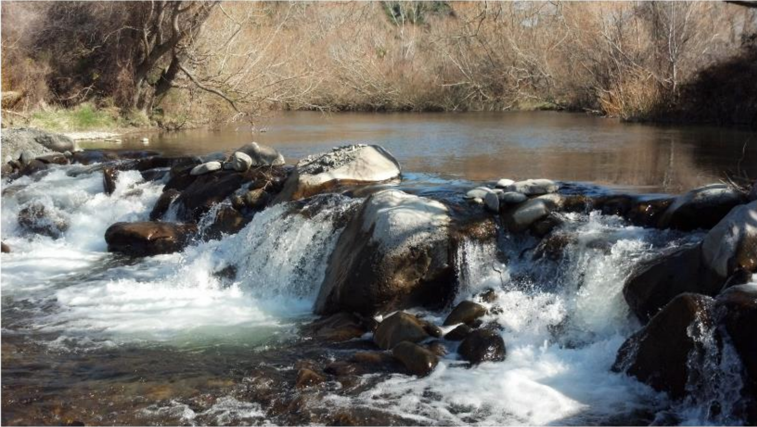
Photo of Selwyn Intake Structure
