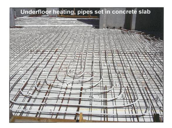
Pipes carrying hot water set into a floor slab is the most common way to do provide central heating as shown in this picture, but largely limited to new houses though is possible for retrofits. (Pipes tied to mesh prior to concrete being poured.)
