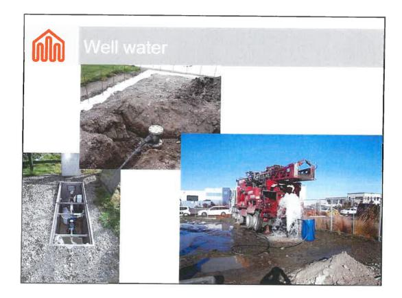
Examples of wells, the right hand picture shows the extract well being drilled for Central Heating New Zealand's new offices which are heated and cooled by a ground water heat pump.
