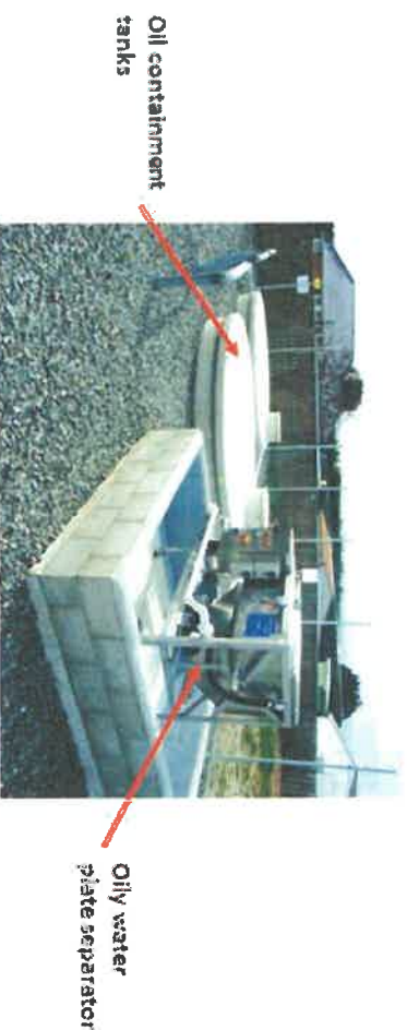
Blenheim Substation oil containment and oily water plate separator system
