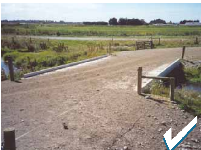
The nib wall on bridge (raised edges) prevents effluent washing into the stream, aided by grass berms filtering the same discharge.
